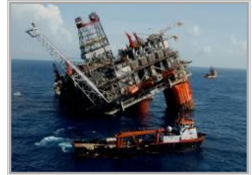
240E class HOS Innovator surveying hurricane damage at BP's Thunderhorse
