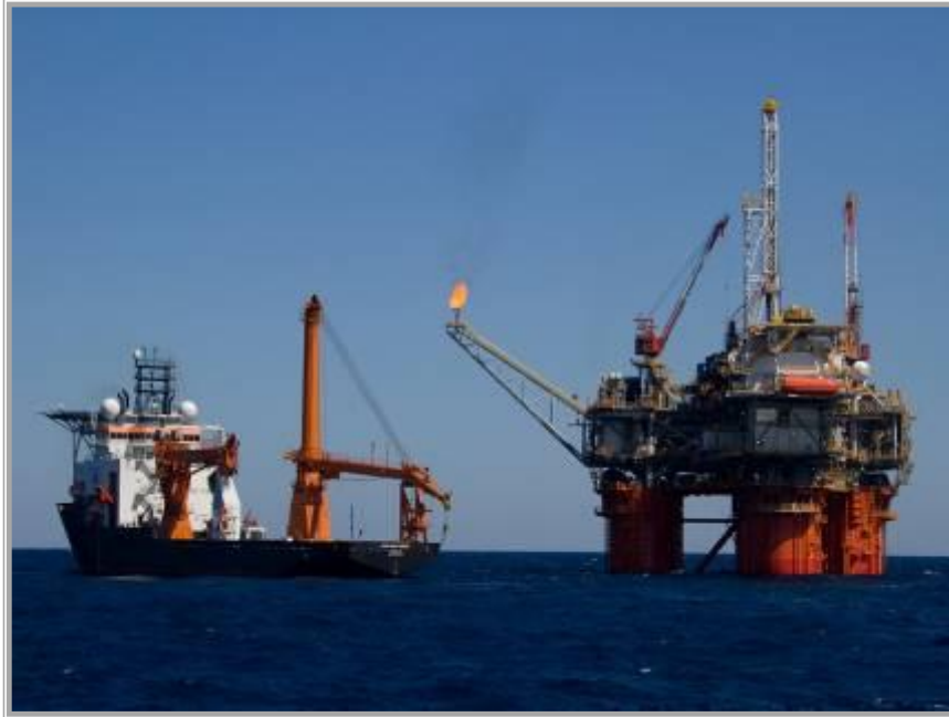
The HOS Iron Horse performing subsea support
