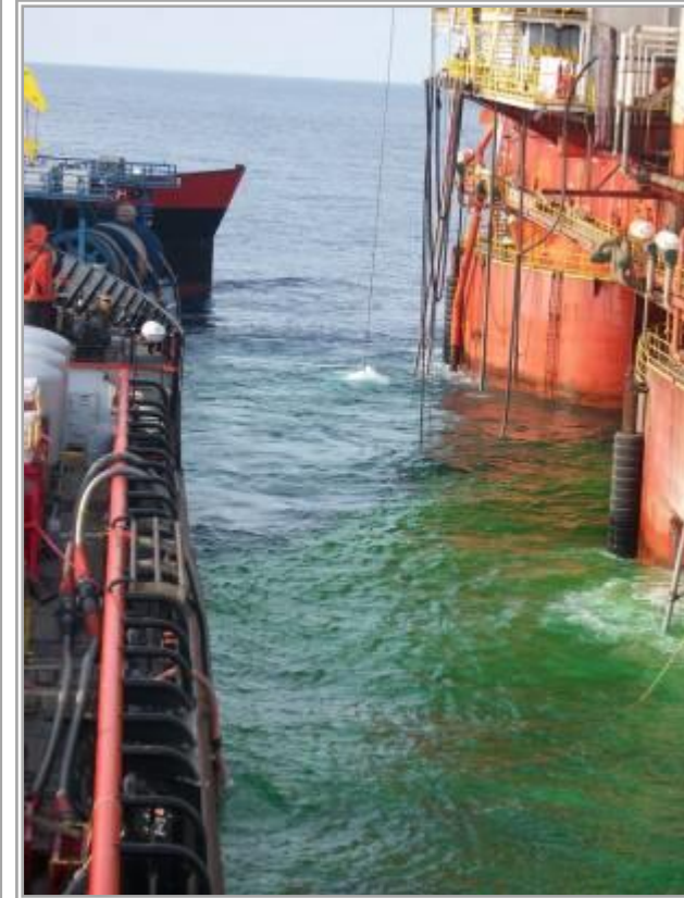
Pumping hoses deployed overboard the HOS Centerline to the Q4000
