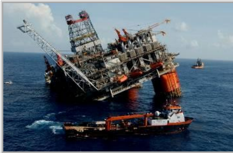
DP2 240E class OSV, HOS Innovator surveying damage at BP's Thunderhorse semi-submersible production platform after Hurricane Dennis in 2005.
