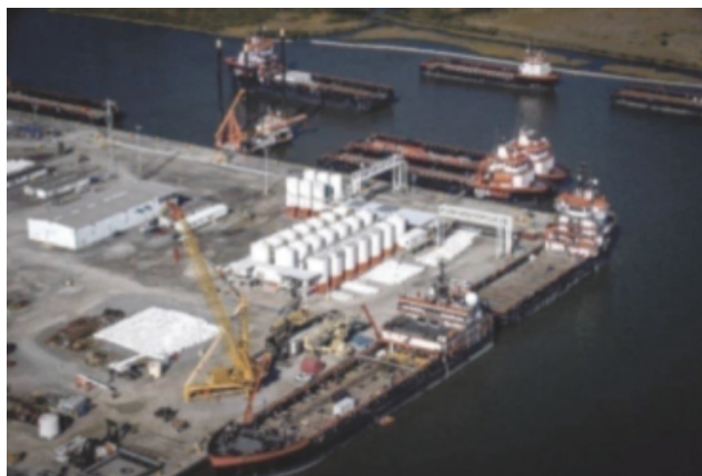
HOS Port Facility in Port Fourchon Louisiana
