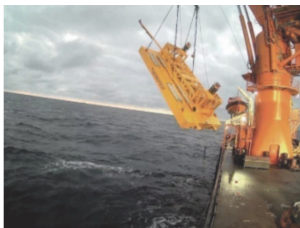
HOS Warland Setting Subsea Equipment
