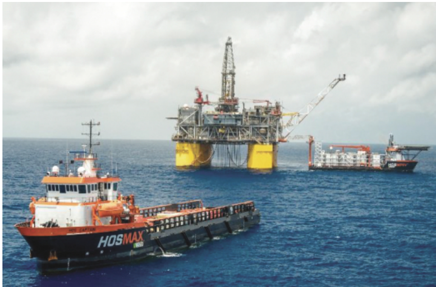
HOSMAX OSV and MPSV flotel servicing an offshore production facility in the U.S. GoM
